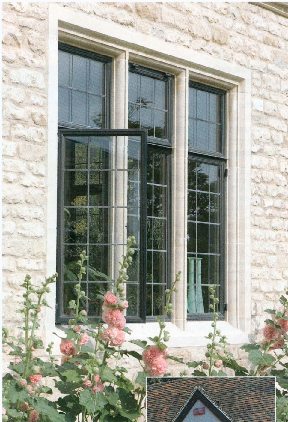
Architectural Bronze Casements — such as these by Vale (ABOVE) — offer a delicate alternative to steel and aluminium — perfect for the detailing necessary to make small panes attractive.
