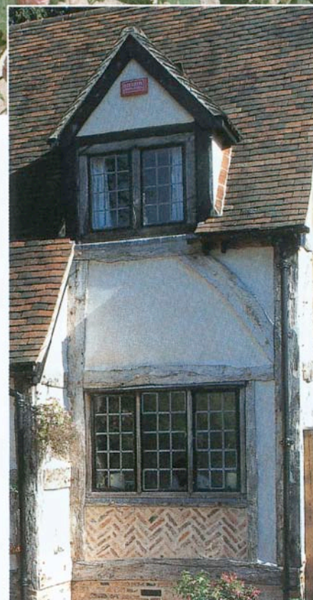
Architectural Bronze Casements — such as these by Vale (ABOVE) — offer a delicate alternative to steel and aluminium — perfect for the detailing necessary to make small panes attractive.
