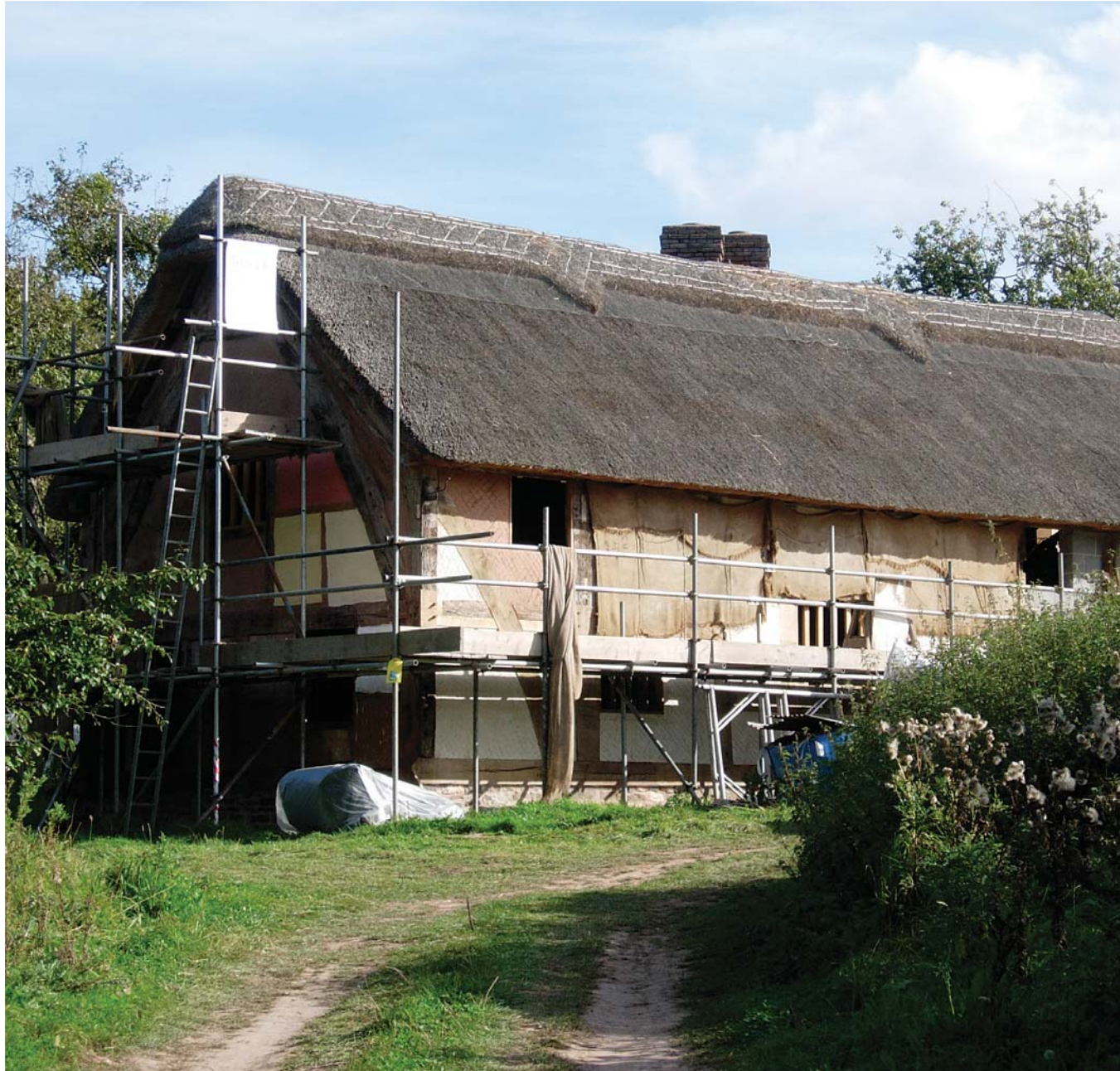
Above: When he was over from New Zealand Phil worked on most of the new wattle and daub infill panels
