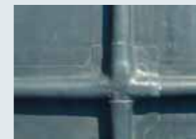
Similar but less complex detail; neatly bossed and looks OK to the untrained eye, however...
