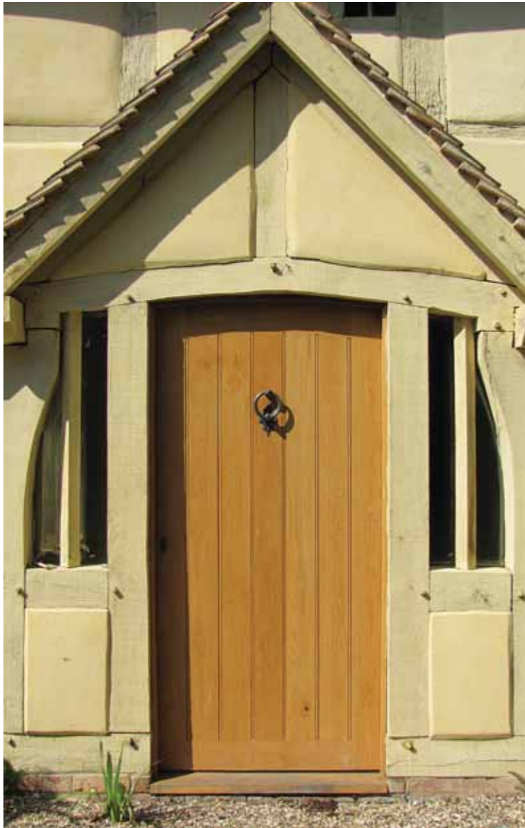
Left: The green oak porch was hugely expensive and built on site. It replaced a rather pedestrian porch built from painted softwood
