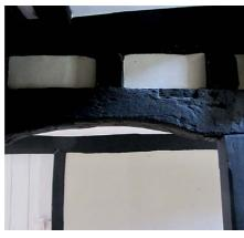
Soon after they moved in Claire and Nick became far more concerned about the rear of the property than the front. When a joiner examined the extension with a view to replacing the windows he found that the bays on both storeys were in danger of collapse
