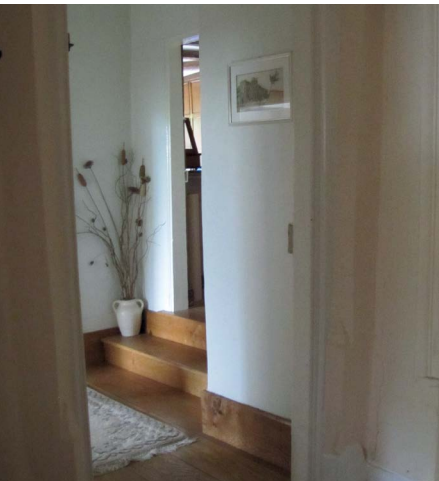
⌵ These steps plus different heights of the doorways possibly indicate that the present east side was at some stage a different structure that was later joined to the main house
