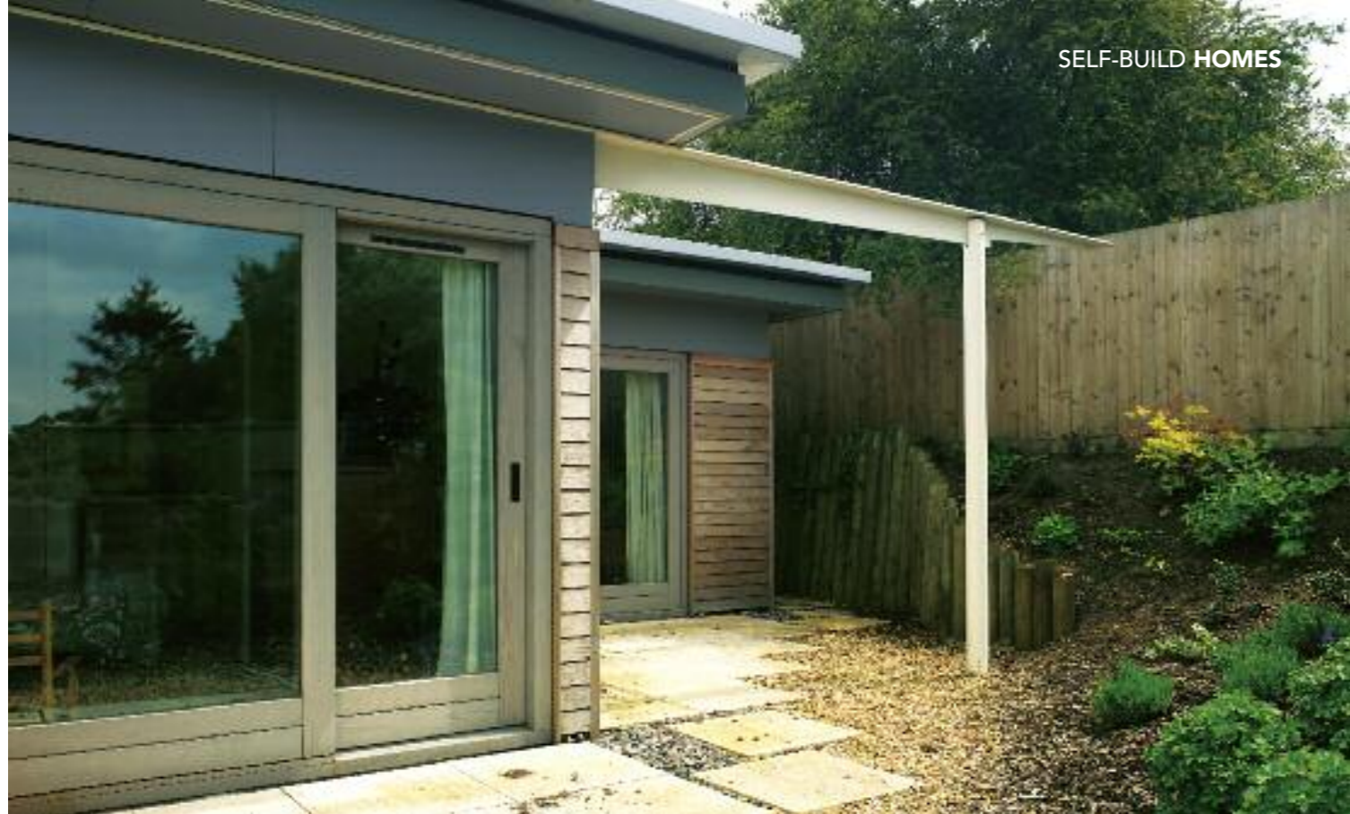
Above: Natural materials meet manmade Cedar cladding is a soft contrast to the hard glazing and structural steel posts. The flat 'warm roof' is topped with a sedum blanket
