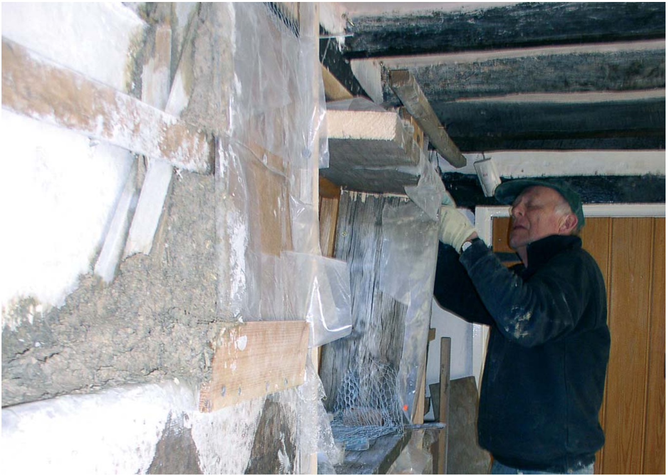
Above: Fixing some of the vertical shuttering
