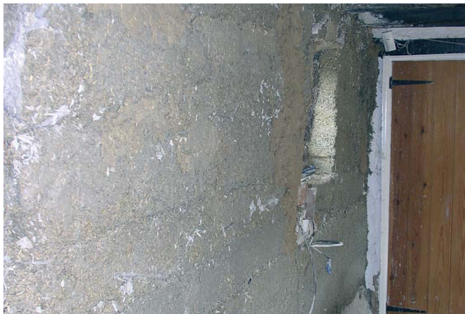
Top left: Applying hemcrete into shuttering round the ceiling beams proved really tricky
