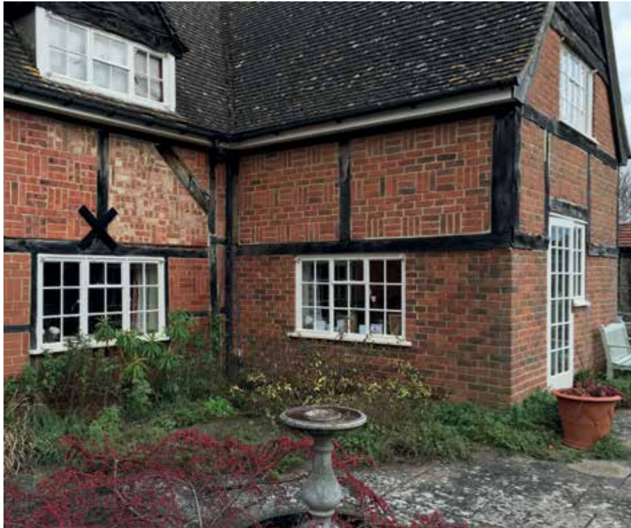
Above left: The 1960s extension can be seen where the timber windbraces end
