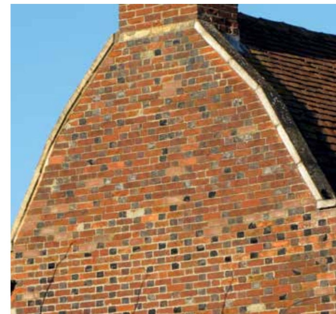
Image 1: This Dutch-style gable end on a house probably dating from the early 17th century has been largely rebuilt. But it has been done well and it is hard to tell from a distance
