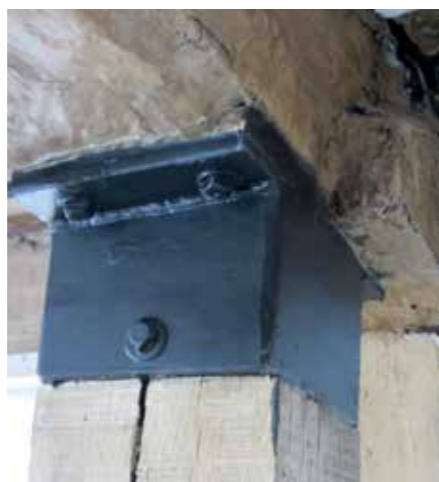
Image 4: These old timbers have been repaired and strengthened where they meet by introducing modern steel. Not advisable – and probably not permissible in a listed building. Inappropriate materials like this usually jar or look downright ugly
