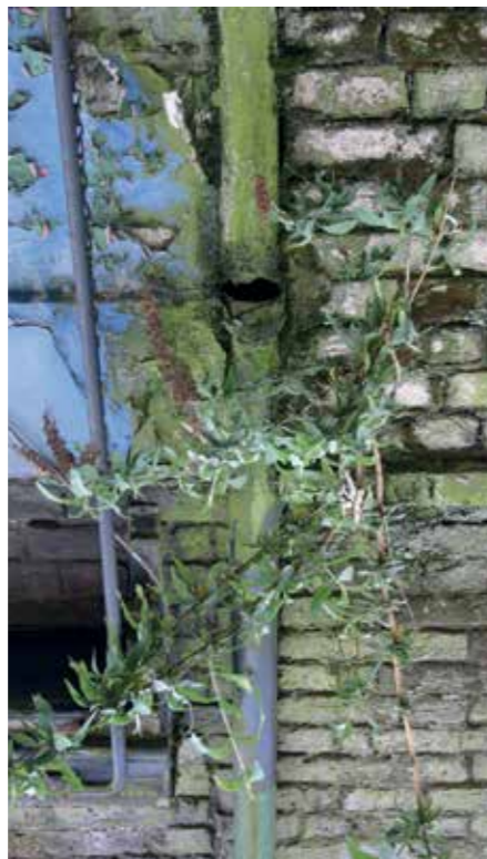
Image 2: Maintaining your gutters and downpipes is vital. If both fail the result can be pretty catastrophic for an old brick wall
