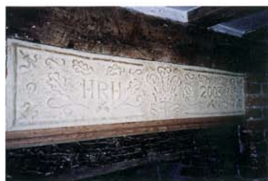
Plastered panels Paula did both these with the normal mix she uses for daub - local chalky clay, straw and water. She did the one with the Prince of Wales' feathers last year to mark an award of £1,000 towards further learning about traditional restoration techniques from Prince Charles' Craft Scholarship Scheme
