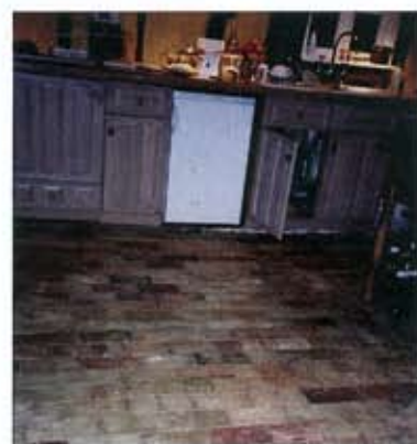
Kitchen floor, laid with a number of reclaimed local bricks
